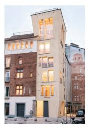
the medieval parts and evoking the former tower system still present in some of the remaining Medieval houses. The project involved the insertion of a new, modern-looking tower that connects the historic façade of the building to the post-
