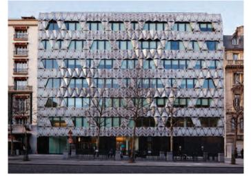
Manuelle Gautrand called this office building on the Avenue Friedland, close to the Place de L'Étoile, the "Origami". The project included two separate parts: a twentymetre long main building along the avenue and an annex behind it, between two gardens. On the avenue, the architect designed a glass façade partially covered by a second layer of glass, which gave it the appearance of folded marble creating a coloured vibration.
