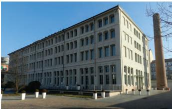
he AC Hotel is located in a former industrial district of the city. The original building was designed in 1908 by engineer Angelo Santonè to host a pasta factory. It was one of the first industrial building in Turin to be built with reinforced concrete pillars and beams. After the damages caused during the Second World War, the building was restored and
