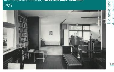
immediately stands out for its planar modernist gualities, designed according to the principles of the De Stijl movement. The interior and furniture, created by both Rietveld and Schröder-Schräder, are an equally integral part of its design. Movable wall partitions created a dynamic open zone rather than a hierarchical arrangement of rooms, which Rietveld and Schröder believed would
