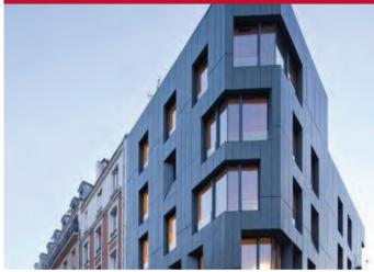
inside" has a railing with an openwork design. It serves two flats per floor, along with a lift that opens onto landings from which the outside can be seen through glass panes. The entire building is covered in dark patina zinc and vertically punctuated by a geometric design based on the lines of the façades and the rhythms and proportions of the openings around it. "We also chose a dark zinc to assertively contain the corner" (Borne, 2013), she explained.
