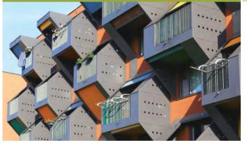
Textile shades provide privacy while still allowing open views over the bay; their strong colours create different atmospheres within the apartments, block direct sunlight and create an 'air buffer' zone. The balcony modules are designed as an efficient system, providing shading and ventilation for the apartments. In the summer, the accumulated hot
