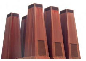
The WKK - Warmtekrachtkoppeling Centrale was designed in 2002 for the University of Utrecht to increase the capacity of two power stations that already existed in the Uithof neighbourhood in Utrecht. Van der Pol designed this building in order to protect the machines and soundproof the building. It is made of weathering steel (Corten steel), which naturally oxidizes and turns the steel into a brown colour. The form of the building becomes a sculpture within the landscape.
