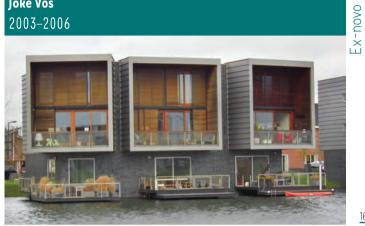
floor and first floor both feature a spacious wooden balcony terrace facing the waterfront. On the wooden platform adjoining the lower terrace, residents can moor small boats. Special attention was given to sustainability, using durable and low-maintenance natural materials, including hard wood and wire netting, filled with natural stone lumps. Thermal insulation
