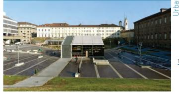
Roberto Gabetti and Aimaro Isola. Two slopes link the central space with the surroundings streets, while the other two form 'wings' covering the parking entrances and ramps. Furthermore, three of the slopes contains green areas, whereas the fourth has stone paving. In the middle of the square a glass building has been constructed, originally designed to house an information
